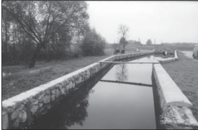
Vibrupe - one of the Latvia's small rivers which has been canalised. Photograph by Janis Brizga
