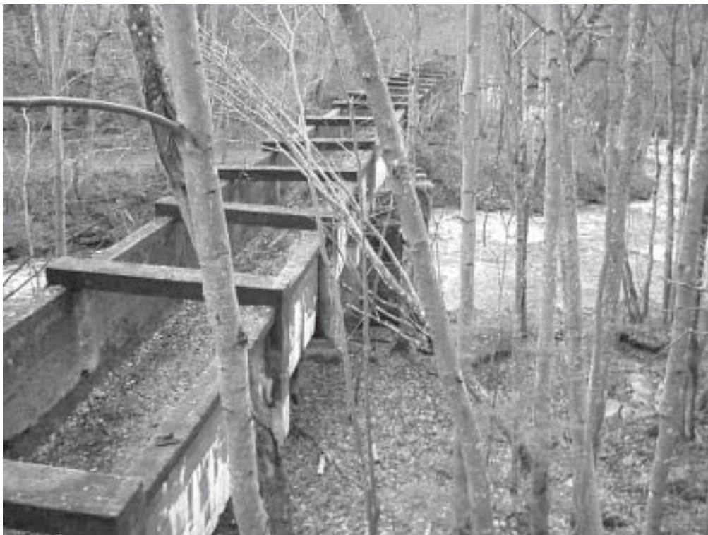
Old derivation channel in previous Nõmmeveski hydropower plant. Photograph by Kaja Riiberg
