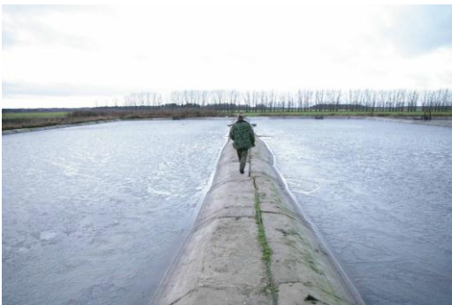
Fig.5. System of consecutive cleaning reservoirs on one of the pig farms, Grodno region
