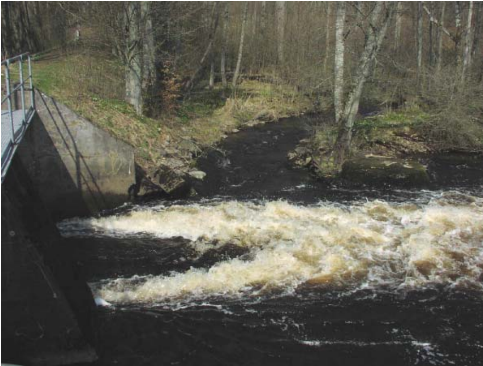
River Alma, Spånga damsite. The opening of the constructed fish way is in the centre of the photo.
